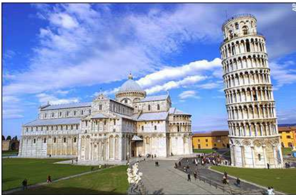
Leaning tower of Pisa, Italy
